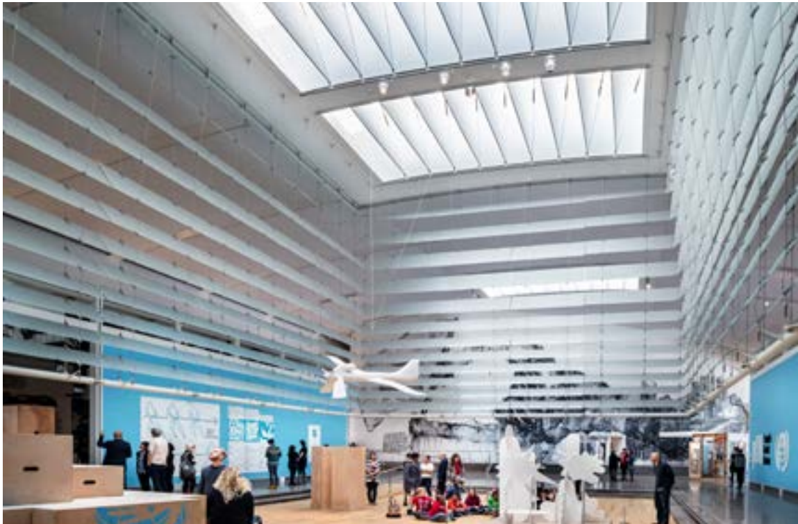
NEW/MIRODAL ACOUSTIC PANELS USING ACM 15 / WHITE MATTE MICRO-PERFORATED MEMBRANE WITH GHOST ROUND TUBE RAIL AND CD TUBES / Z-CLIP SYSTEM.
