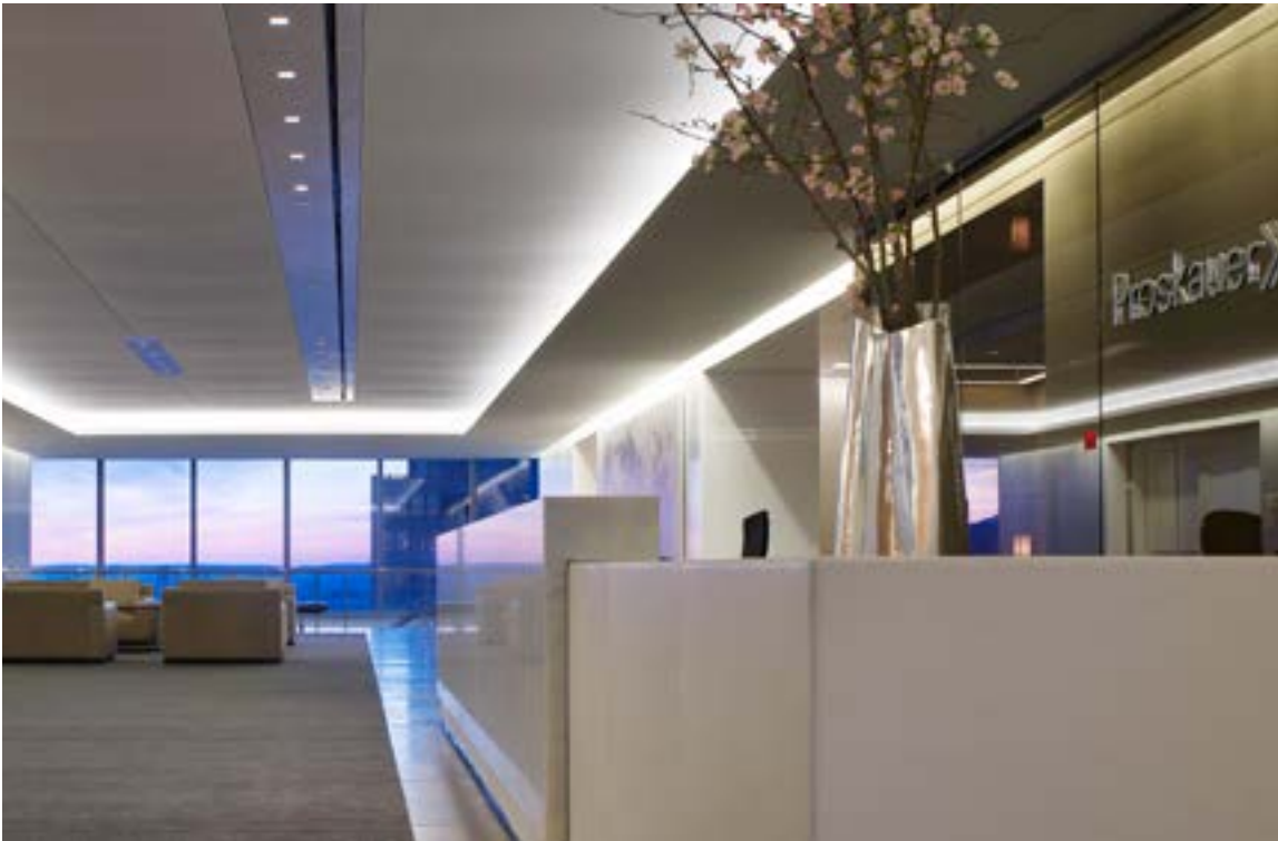
NEW/MIRODAL CLASSIC PANELS USING M15 / WHITE MATTE MEMBRANE WITH SOUND REFLECTOR BACKING / CUSTOM T-BAR GRID SYSTEM.
